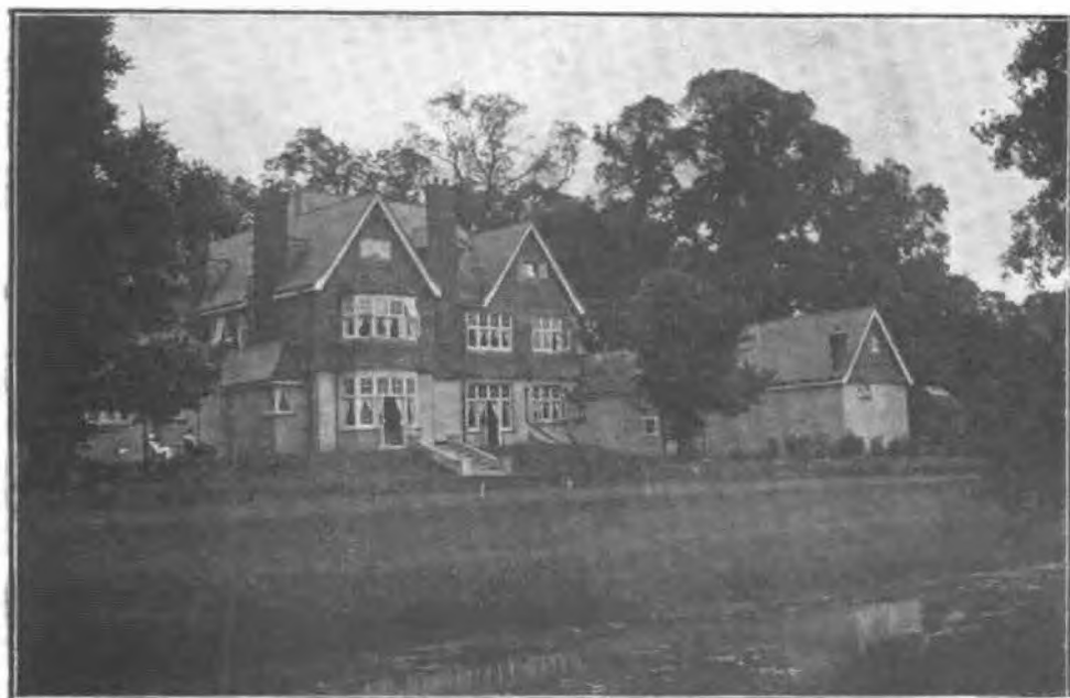
GROVE COURT. VIEW FROM THE GARDEN.
